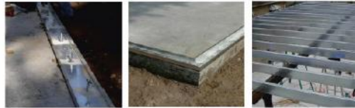
Panels can be installed on a slab or an elevated floor system
