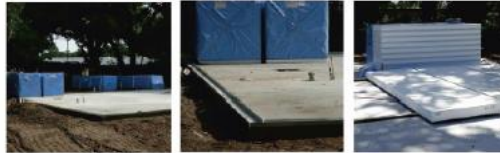
Panels can be installed on a slab or an elevated floor system
